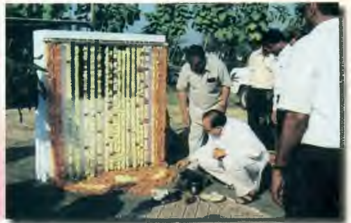
Shri Ranjit Deshmukh, Minister of Agriculture, Govt of Maharashtra State laying the foundation stone of ATIC building.
