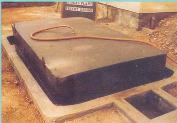
Semicontinuous Biogas Plant
